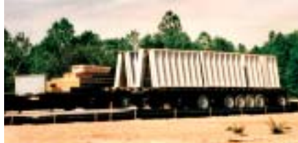
Photograph 10 Pre-cast basement walls
