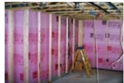
Photograph 8 Unfaced extruded polystyrene against basement wall
