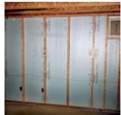
Photograph 9 Unfaced extruded polystyrene against basement wall
