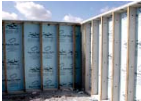
Photograph 11 Pre-cast basement walls with XPS foam insulation
