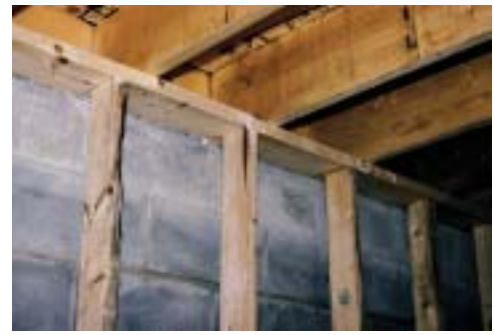
Photograph 1 Interior stud framing located at basement perimeter
