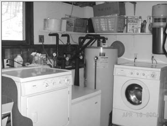
Figure 9.1: Front-loading washing machines can save tens of thousands of gallons of water and hundreds of dollars over their lifetime.
